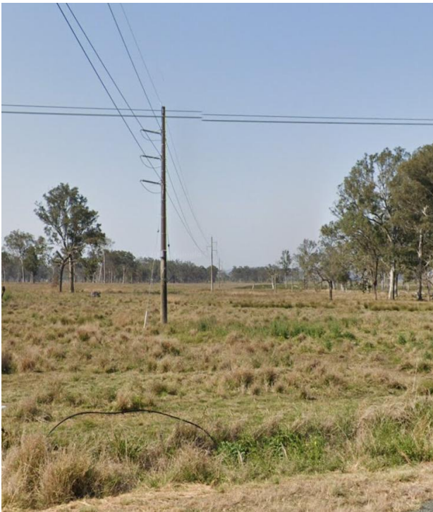
Figure 6: Example of existing overhead powerlines
