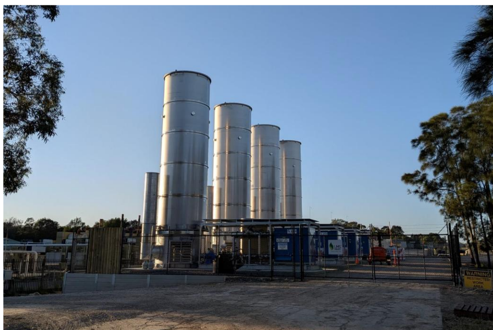
Figure 6. Installation and commissioning of 5x new flares and 2x temporary flares
