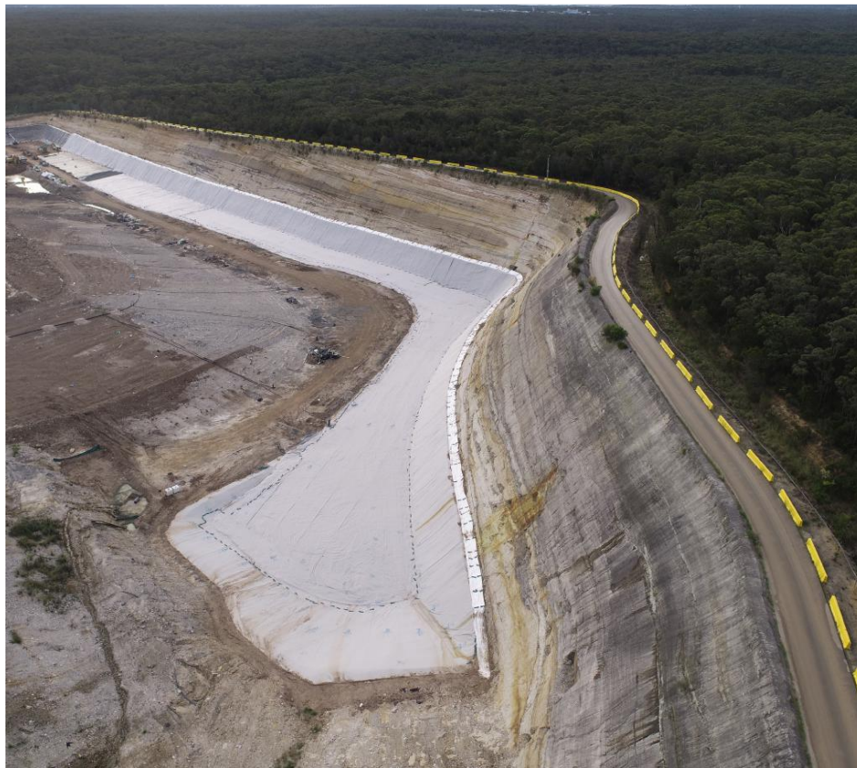
Figure 2. Liner installation at the North Wall Area
