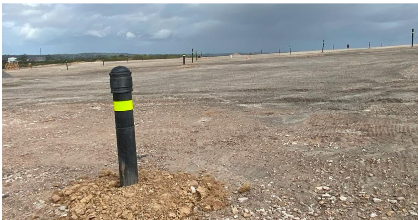
Figure 4. Installation of gas collection wells at Area C.
