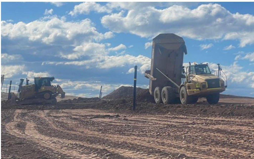
Figure 5. Capping works in Area C
