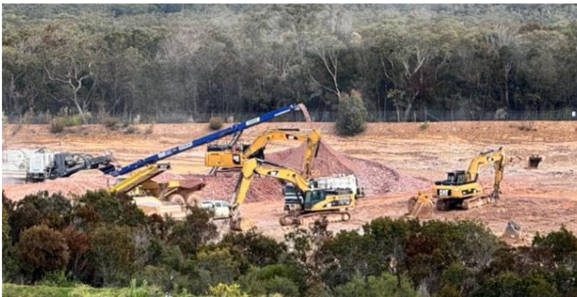
Figure 3. Stage 2 excavation at the proposed western Garden Organics area
