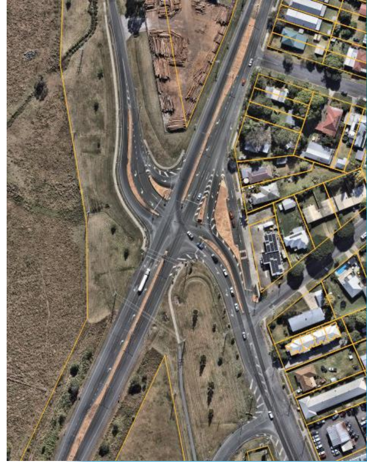
Beaudesert Bypass Road / Mt Lindesay Highway / Brisbane Street / Helen Street signalised intersection
